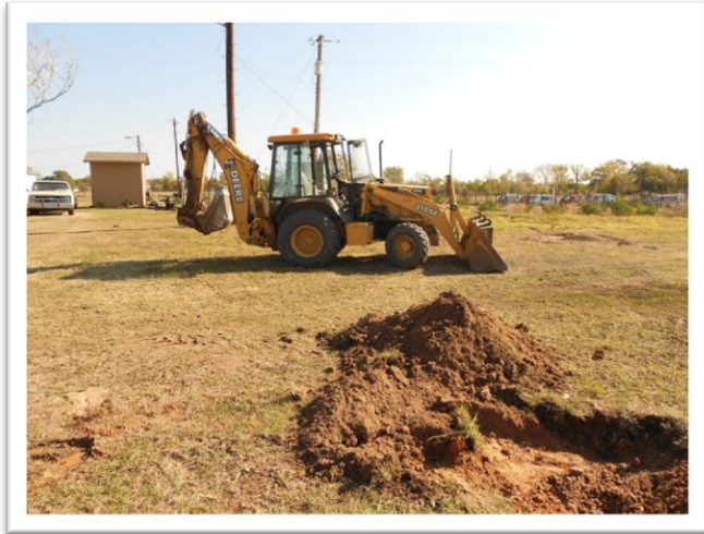
PICTURE 1: GAS TANK CONSTRUCTION
