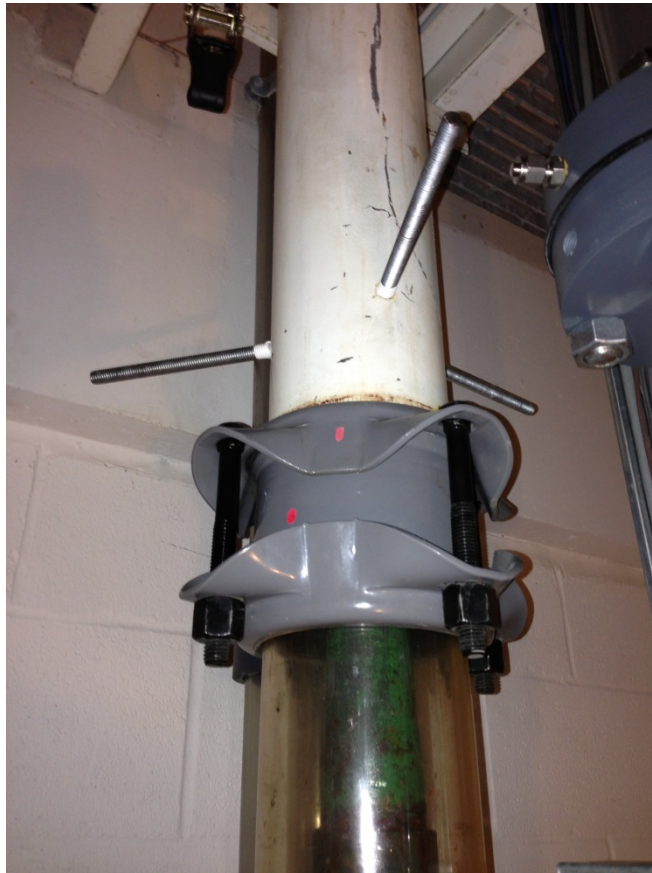
Figure 9: Detail of the positioner with its three screws.
