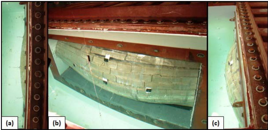
Figure 5.73. SW20. (a) Deformation passed the frame. (b) Vertical and horizontal cracks on wall continued to expand. (c) Gauge D1 disengaged from film surface. (Adapted from Johnson, Davis, Coltharp, Durst, and Smith 2010)
