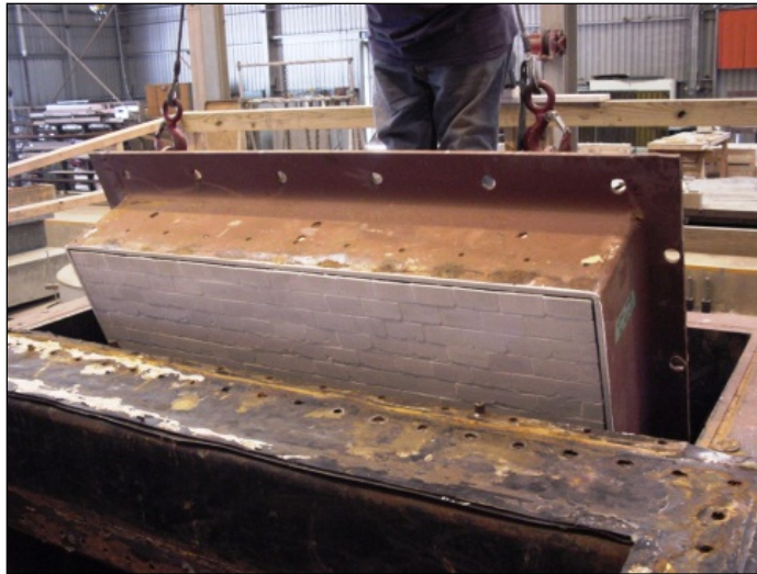
Figure C30. Lower wall frame into position.
