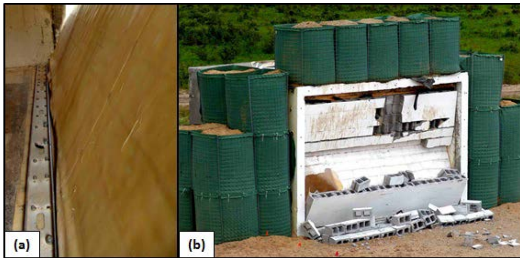
Figure 7.34. FS10. (a) Bottom support was engaged during wall response. (b) Hours after the blast event, the bottom section of the wall disengaged from the retrofit material.
