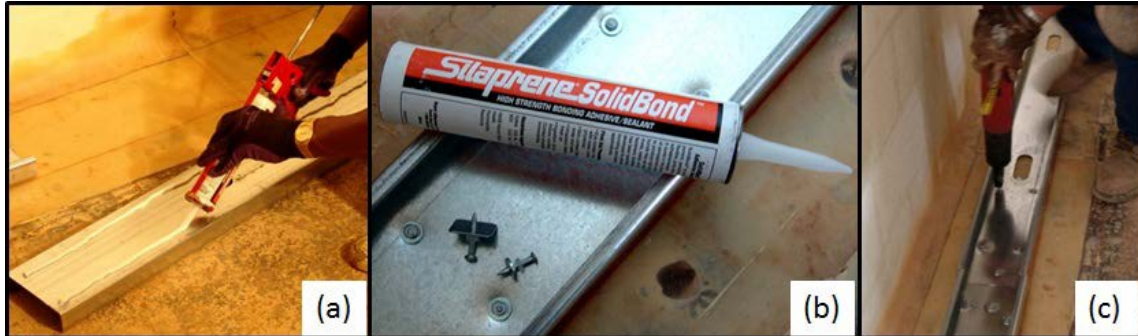
Figure 4.16. Anchor System 8. (a) Steel stud member. (b) Adhesive. (c) Ramset and nails required for installation.
