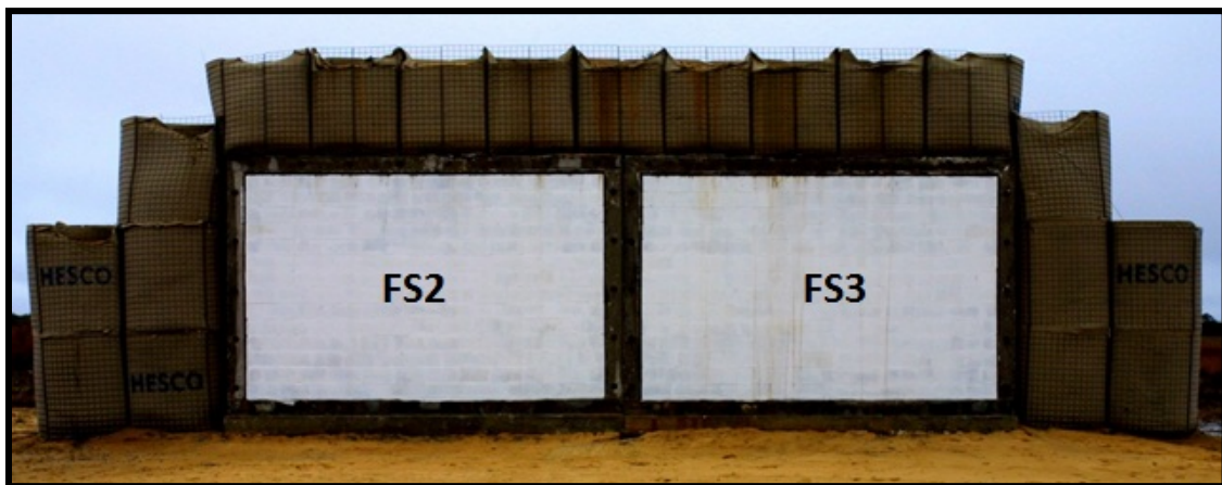
Figure 7.8. Pretest photograph of walls FS2 and FS3.
