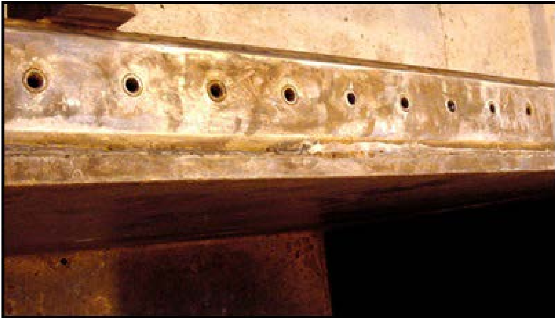
Figure C16. Cleaned side walls of pressure cavity.
