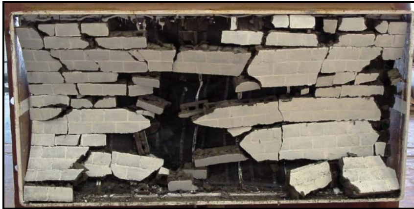
Figure 5.63. Damaged CMU blocks and area where the blocks lost adhesion.
