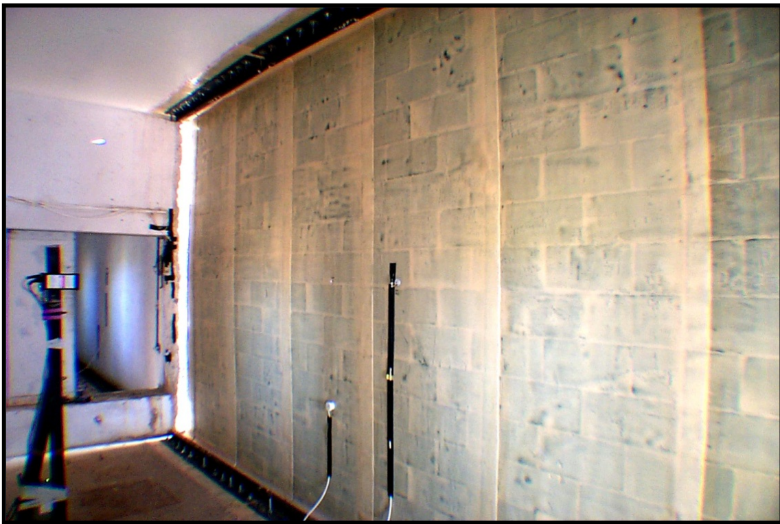
Figure 4.55. Each successive sheet overlapped the previous sheet.
