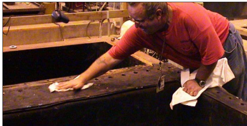
Figure C4. Neoprene seal is cleaned prior to application of new silicone.
