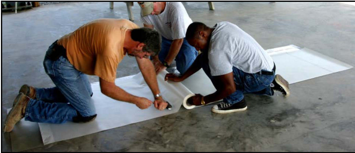
Figure 4.64. Acrylic adhesive applied to the elastomeric film in the field.
