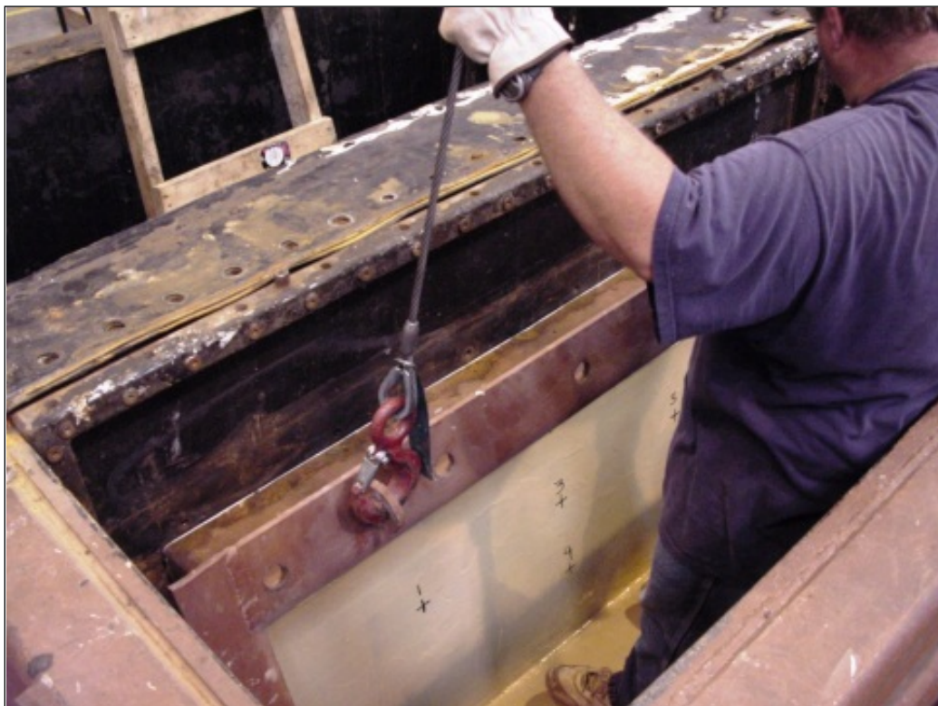
Figure C31. Technician counter balances frame to lower the wall into the chamber.
