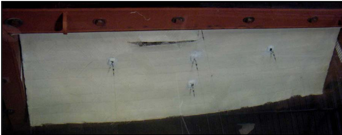
Figure 5.23. Ultimate failure of the retrofit occurred when the materials tore along the bottom anchor plate.
