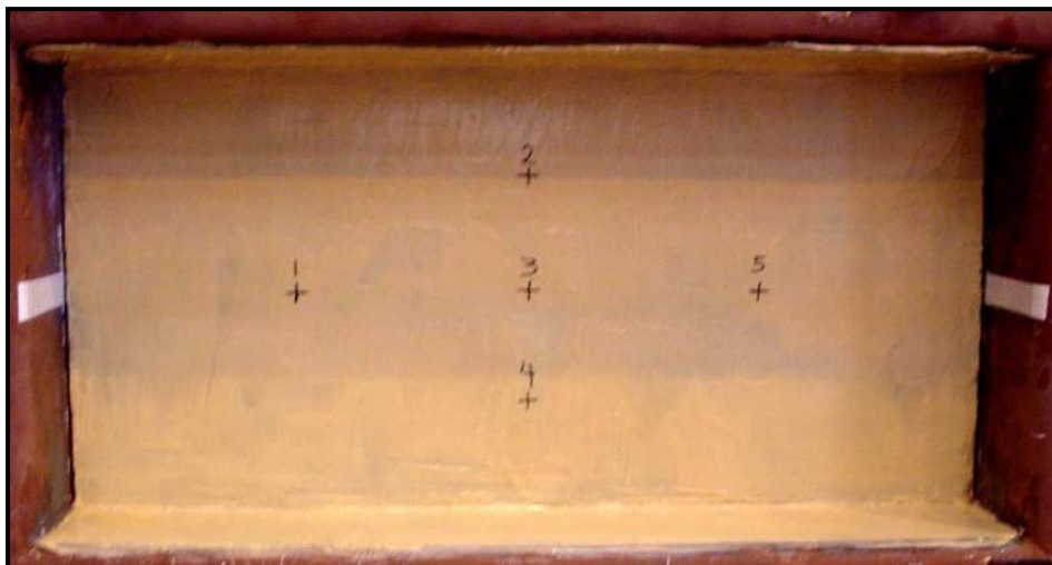
Figure 5.35. SW10 retrofitted with trowel-on thermoset.
