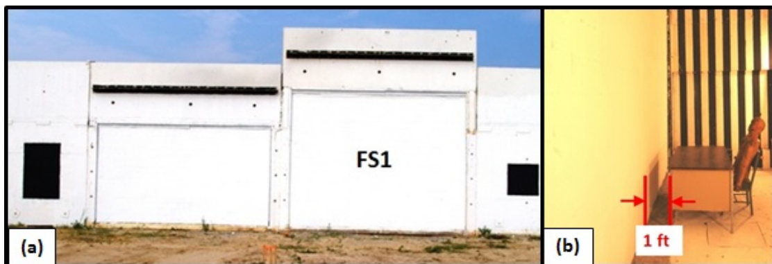
Figure 7.4. FS1. (a) Pretest view of exterior. (b) Interior view.
