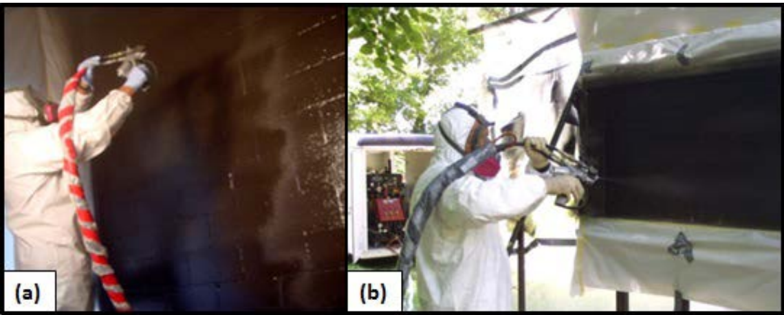
Figure 4.27. Spray-on polyurea. (a) Spray wall surface in a continuous manner until desired thickness achieved. (b) Application of spray-on polyurea to subscale specimen.
