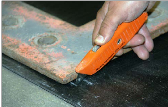
Figure C6. Simple work knife used to cut neoprene material to correct size.
