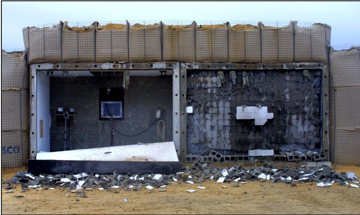
Figure 7.11. Posttest photograph of walls FS2 and FS3.
