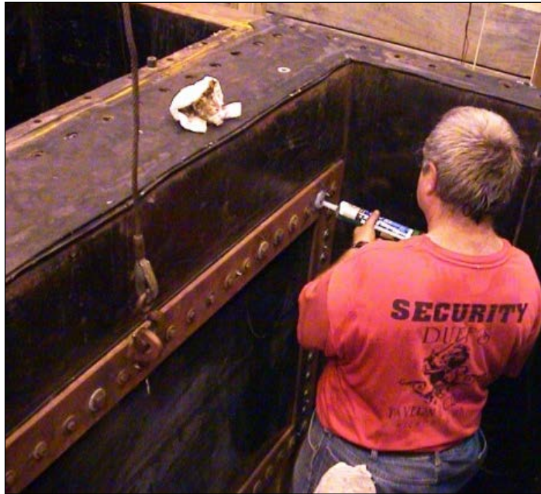
Figure C13. Silicone around bolts that may be stripped.
