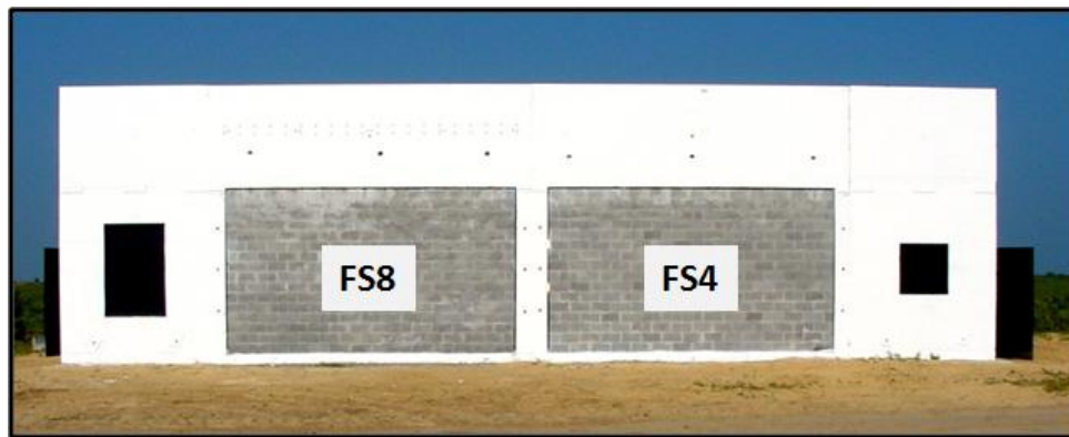
Figure 7.14. Pretest exterior view of retrofitted CMU walls FS4 and FS8.
