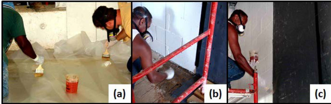
Figure 4.56. Primer application. (a) Prime the film. (b) Prime the support. (c) Prime the 4-in. area on the previous sheet of film that will be overlapped by new sheet.
