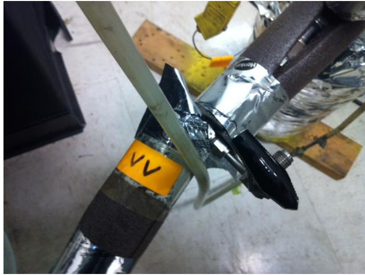
Figure D-7: VV Valve in the CLOSED Position before Changing Aggregate
