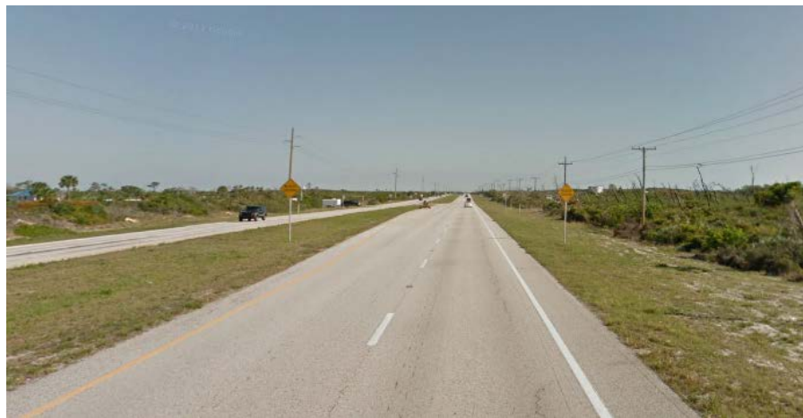
Figure 40 Current view of section 12-0505 in Martin County, Florida.
