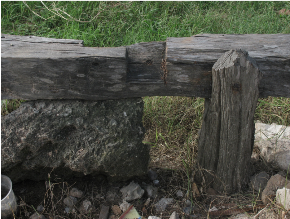
Fig. 5.24. Foundation construction features at the Old Barry House.
