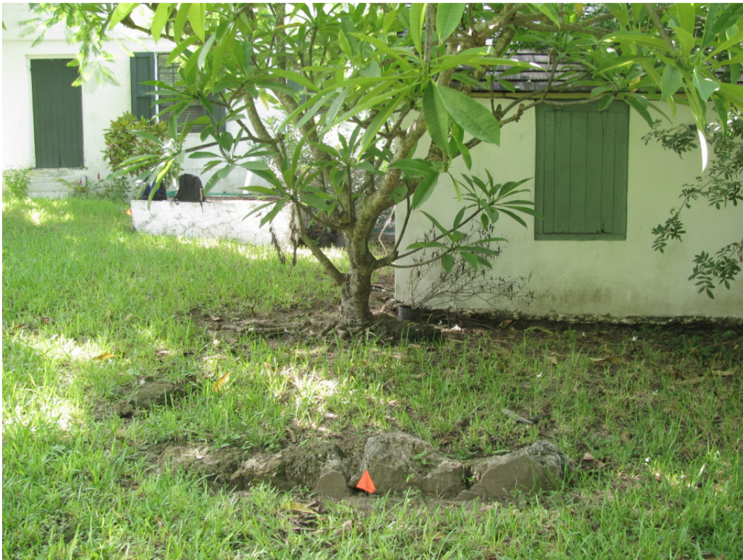
Fig. 5.21. Outbuilding foundation at Methodist House, facing south.
