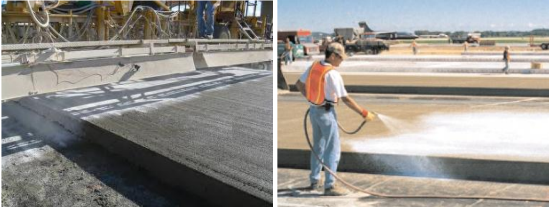
Figure 2-5 Application of curing compound on concrete pavement [3, 20]
