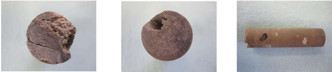
Figure 104: Core 2 Inlet, Outlet, and Side View
