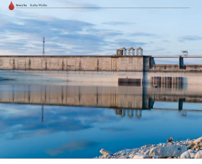
The backside of Mansfield Dam on Lake Travis clearly shows the effect of drought with the water level low enough to expose turbine intakes.
