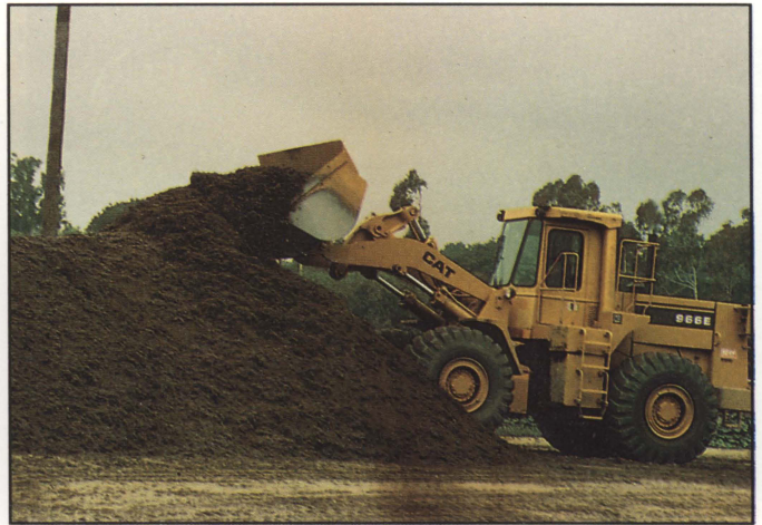
▲ Figure J-2. A conventional front end loader being utilized in a mesh-root zone mixing operation on a hard surface.
