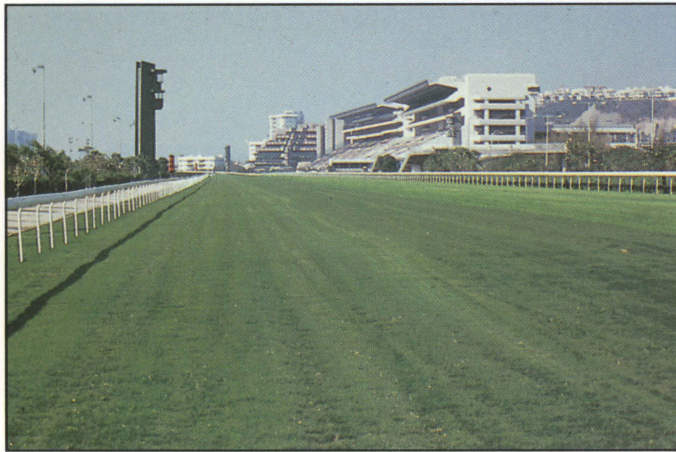
▲ Figure K-1. Sha Tin horse race track in Hong Kong, installed in 1989.
