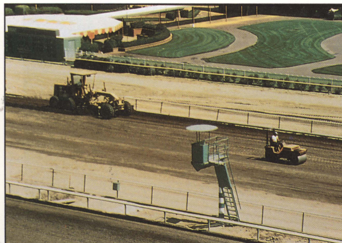
▲ Figure J-5. A power roller and road grader executing the final leveling operations on a moist mesh element high-sand root zone matrix.
