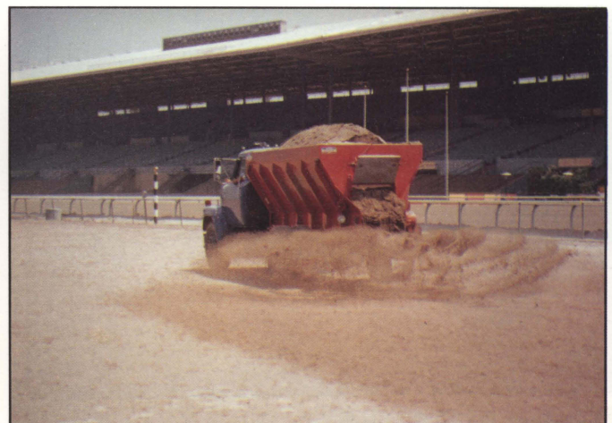
▲ Figure J-6. A centrifugal distributor unit mounted on the back of a truck that is being utilized for application of the 25 mm (1 in.) topdressing.
