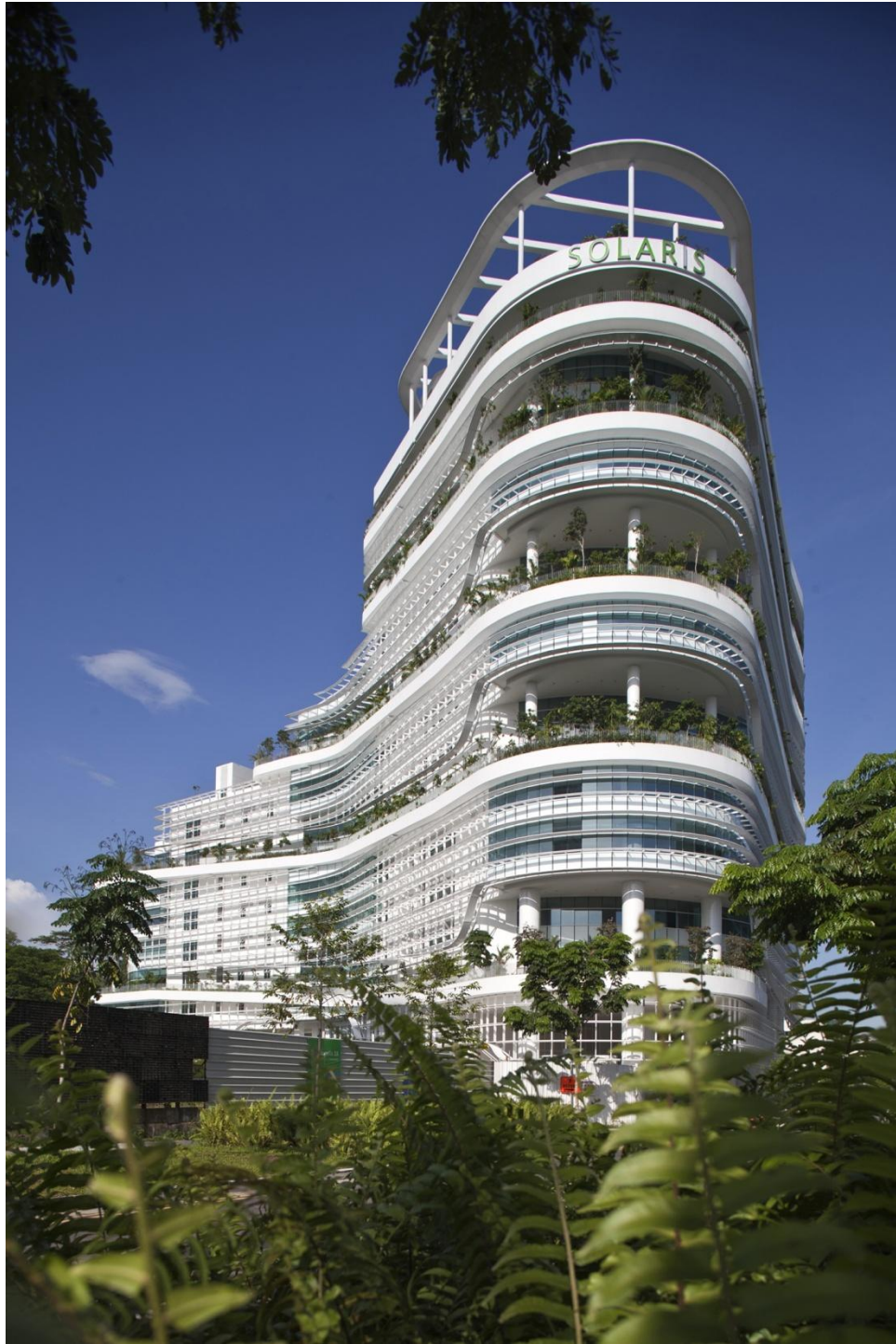
Figure 15: Solaris exterior view (Copyright T. R. Hamzah & Yeang Sdn. Bhd. 2012).
