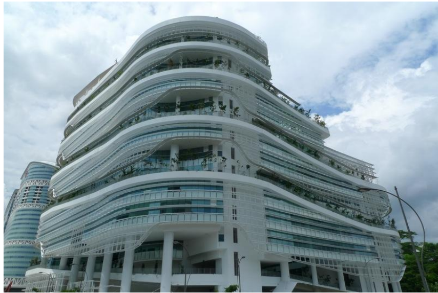
Figure 14: Solaris façade (Copyright T. R. Hamzah & Yeang Sdn. Bhd. 2012).
