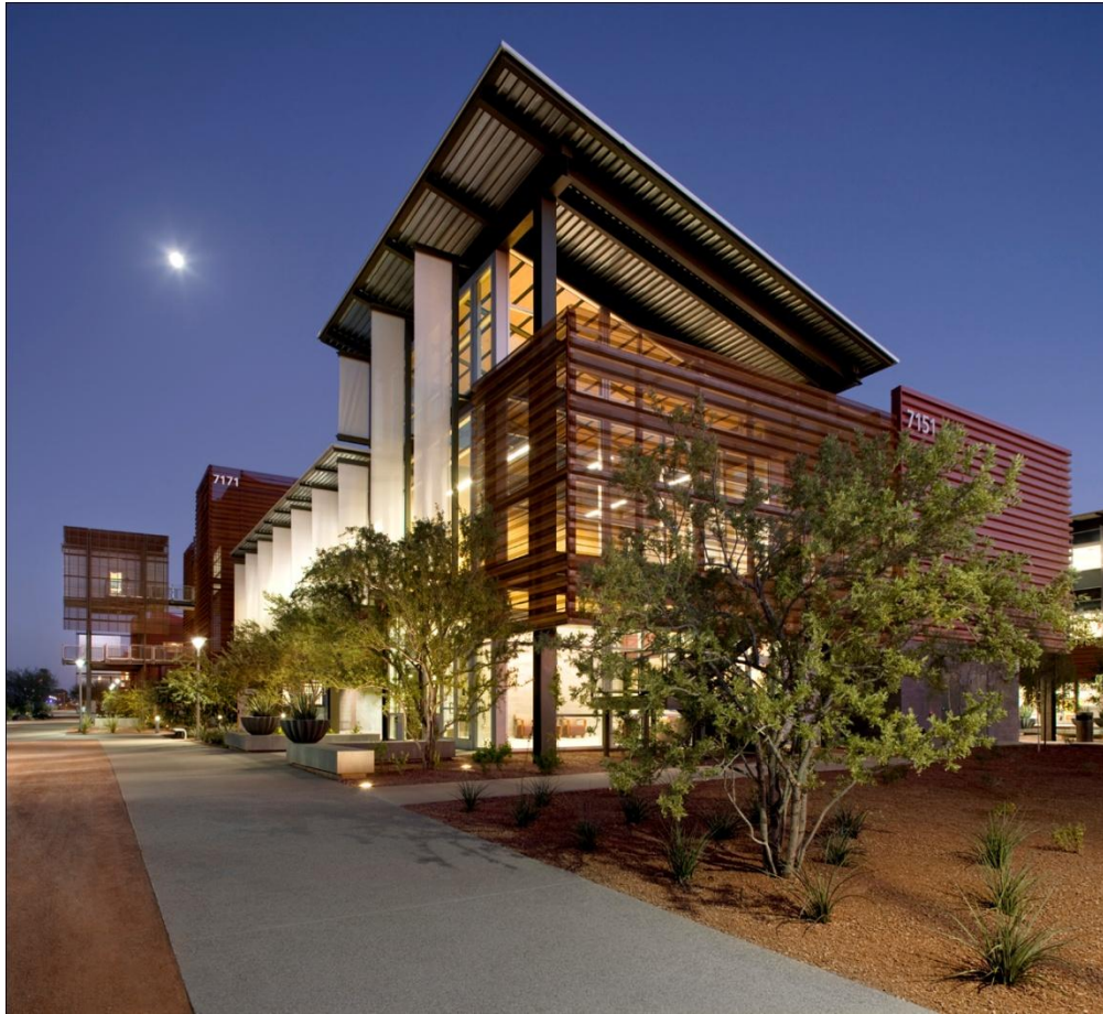
Figure 8: Access to Arizona State University Polytechnic Campus, photo by Bill Timmerman.
