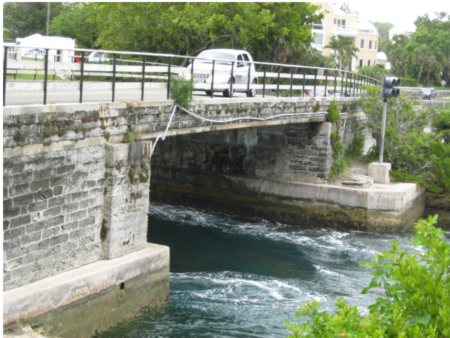
Fig. 1.4. Water flowing under Flatts bridge during a falling tide.
