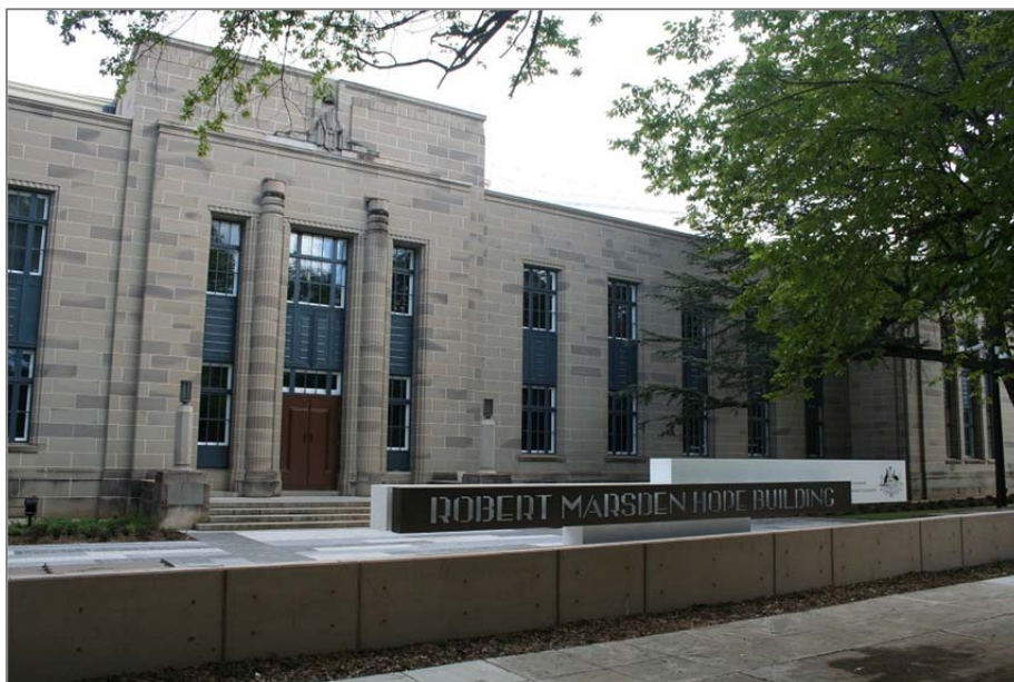
Fig. 2. Sandstone façade, heritage listed office building – Canberra Australia
