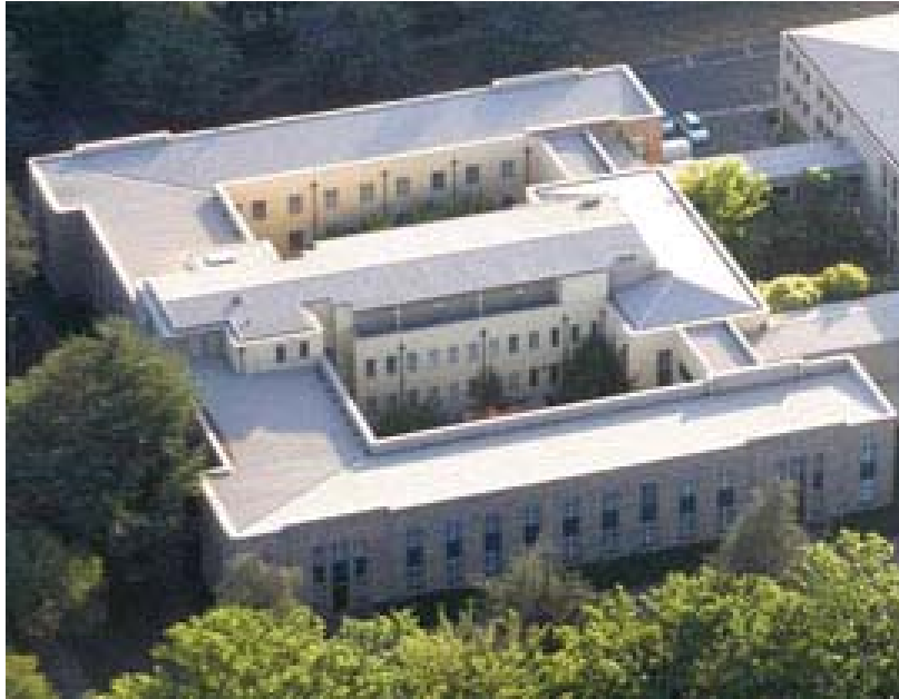
Fig. 1. Aerial view of 2 National Cct office building – Canberra Australia
