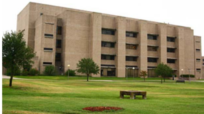
Fig. 2. Case study building
