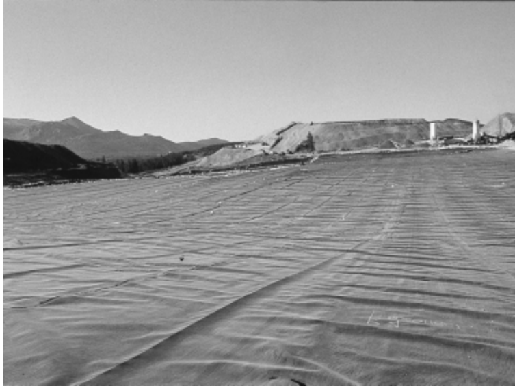
Figure 1.1 Construction of heap leaching pad at Pikes Peak, Colorado, USA (Logsdon 1999)
