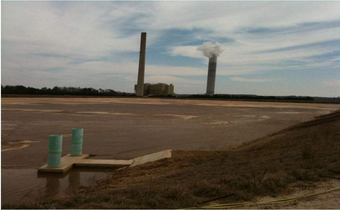
Fig. 6. FGD Settling Pond at Plant Wansley, Carrollton, GA
