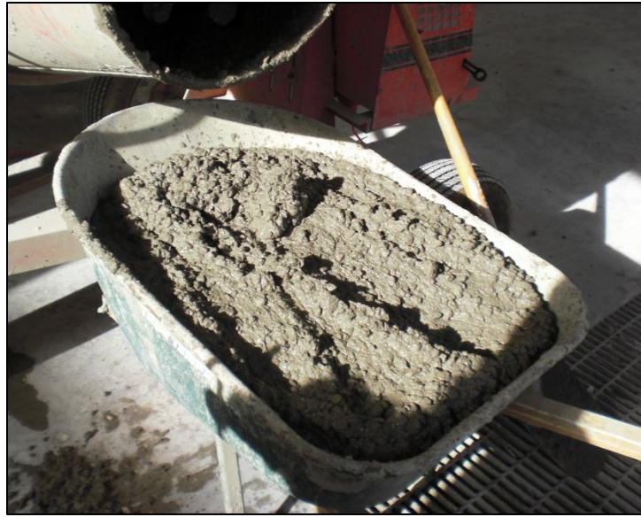
Figure 4.2. Fresh concrete after pouring from mixer.
