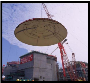
Figure 39 Installing the dome module of NPP (IAEA, Advanced construction methods for new nuclear power plants, 2012)
