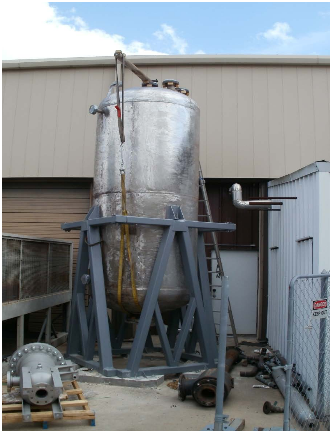
Figure 4.2 Rear of tank showing the temporary crane arrangement
