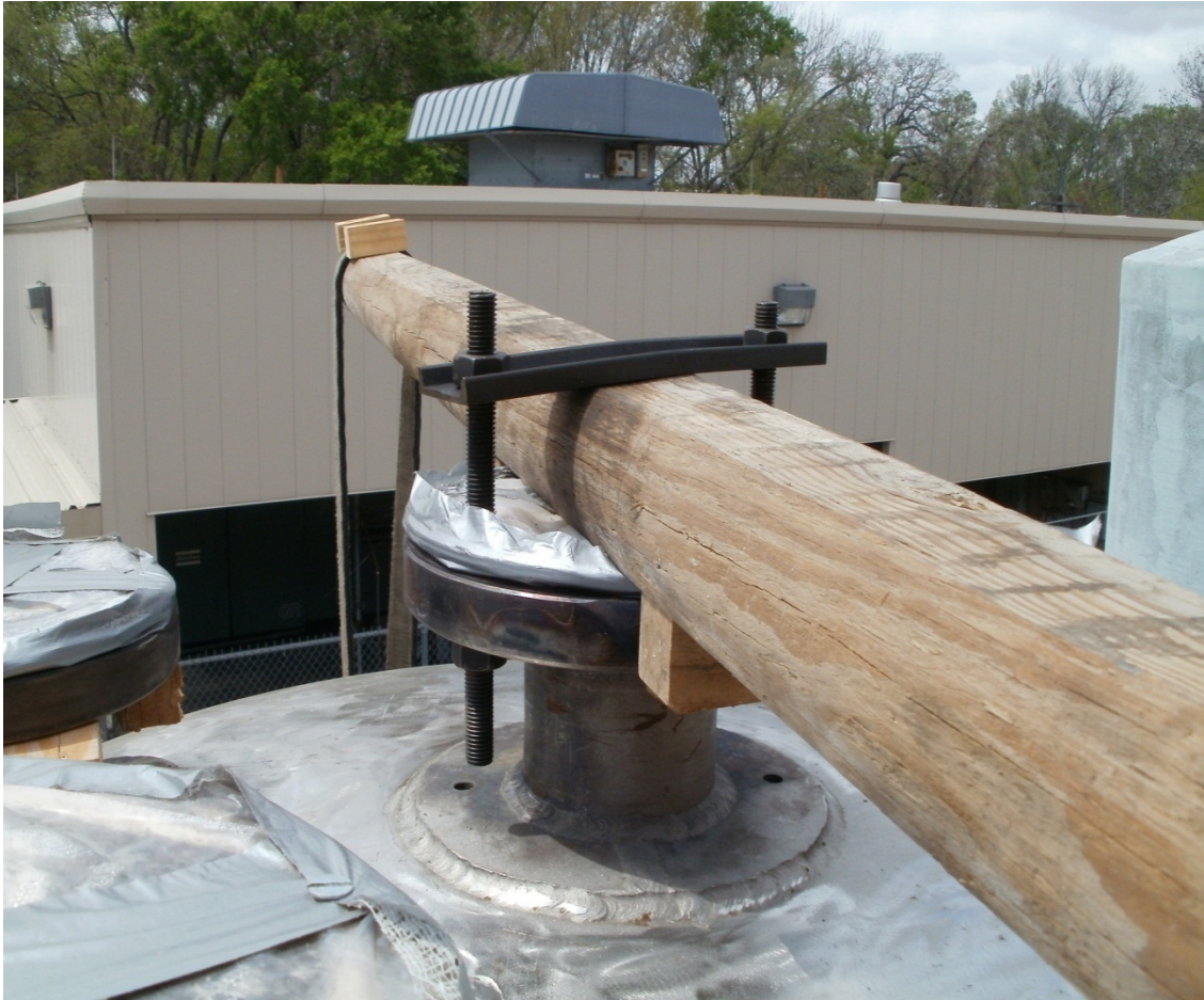
Figure 4.3 Temporary crane assembly mounted to top of separator tank
