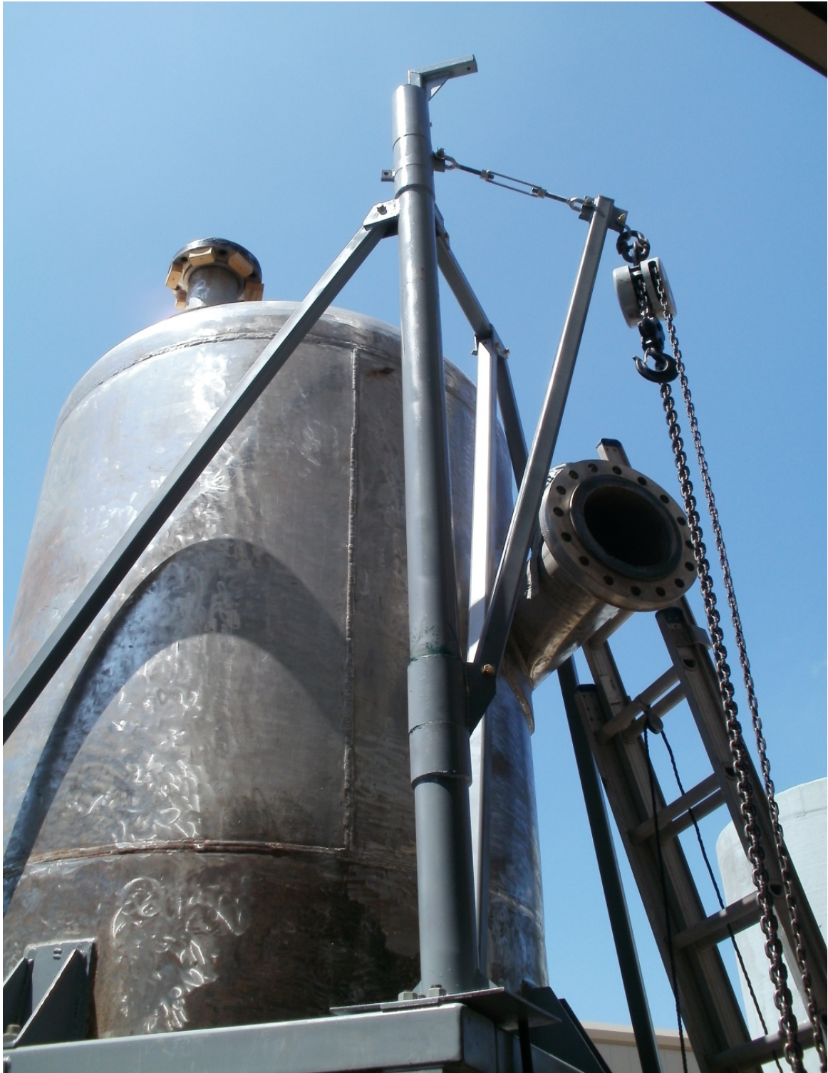
Figure 4.4 Ready to lift spool seven
