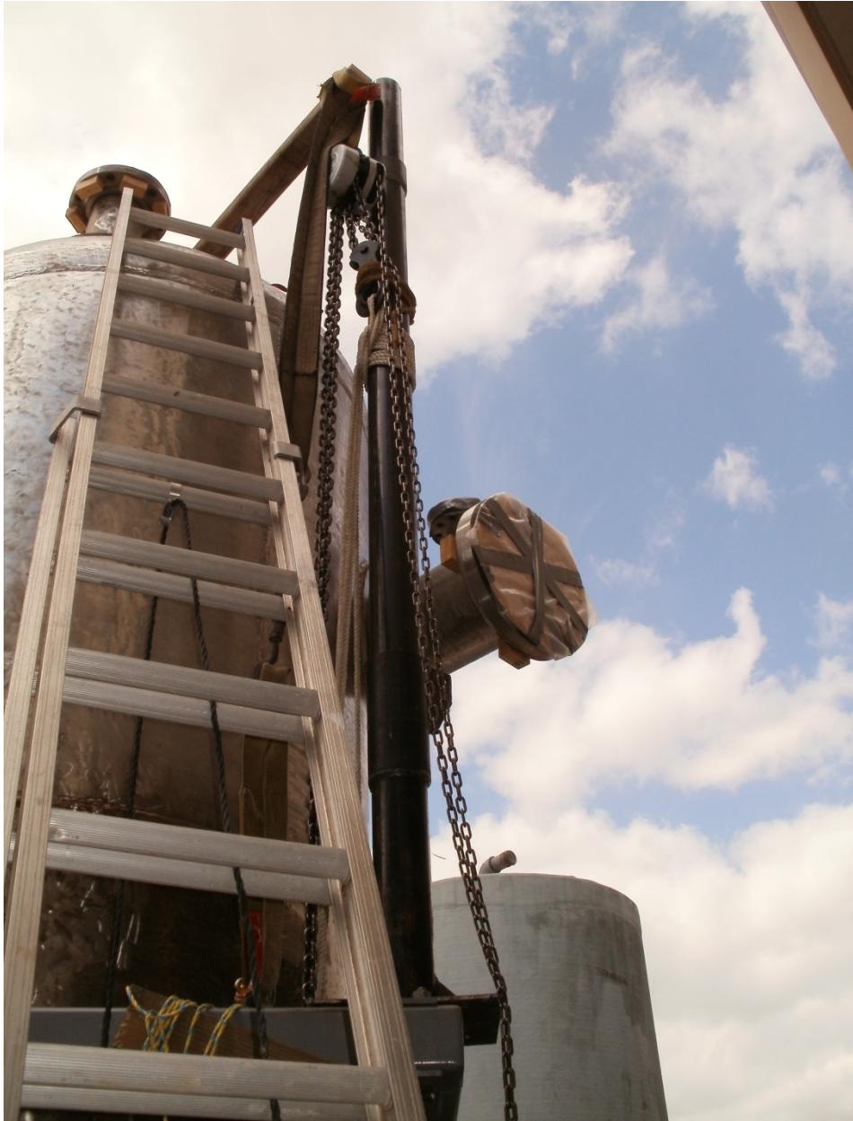
Figure 4.1 Main support column being raised
