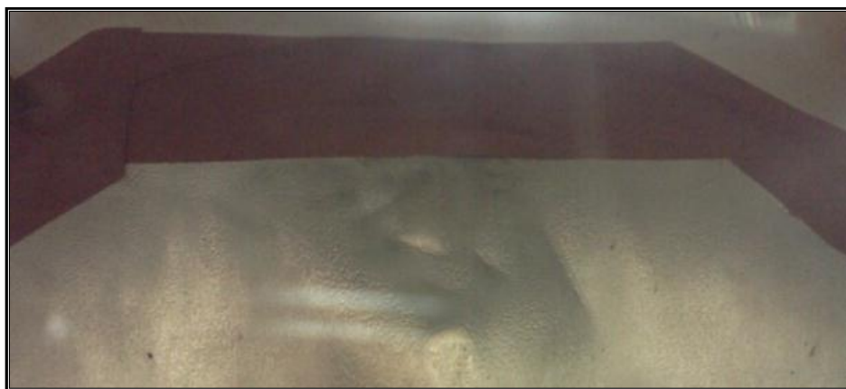
Figure 3-24: The silicon anti-friction tape over the joints inside of the catch pan.
