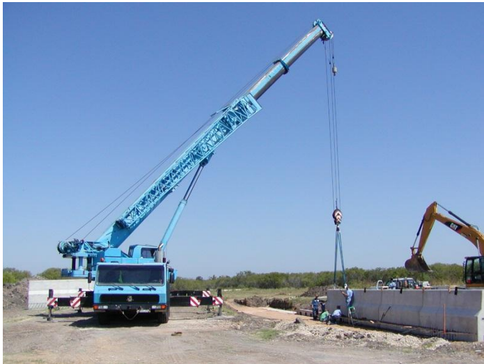
Figure D.13 Installation of the TL-5 precast concrete barriers
