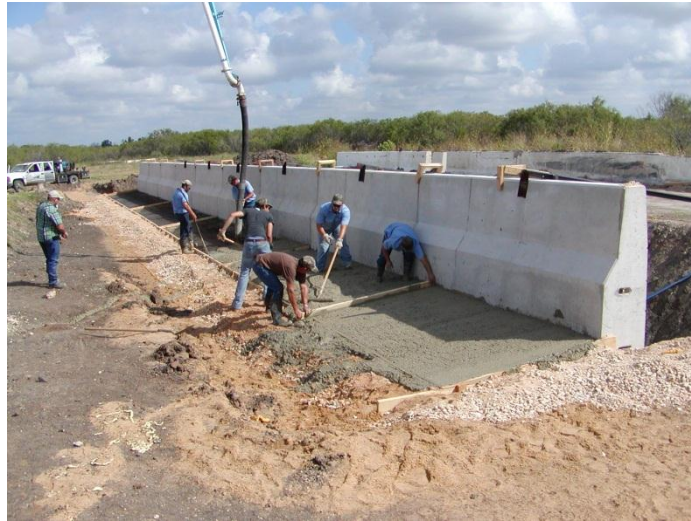
Figure D.15 Construction of the moment slab sections
