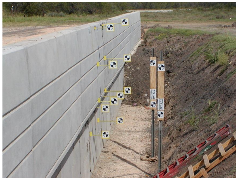
Figure 7.34 Location of displacement bars affixed on the barrier and panels.
