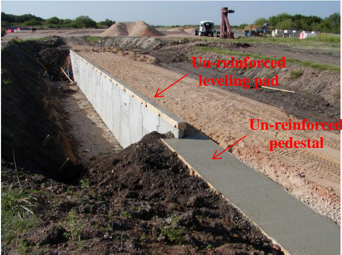
Figure D.11 Un-reinforced leveling pad and pedestal
