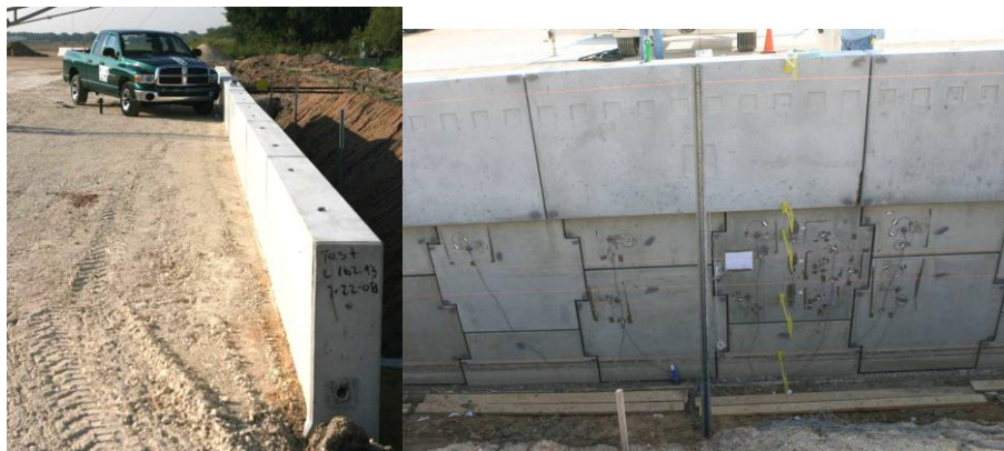
Figure 2.12 Barrier on MSE wall prior to testing (2)
