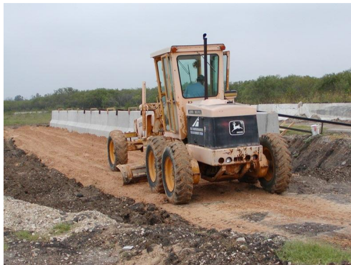
Figure D.16 Placement of road base material above the moment slab
