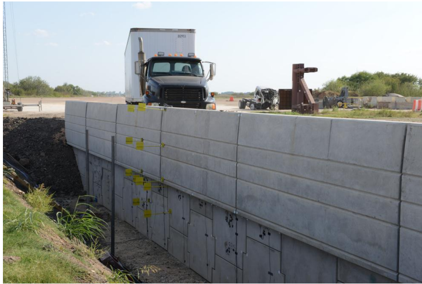
a) Full-scale MSE wall and vehicle set-up
