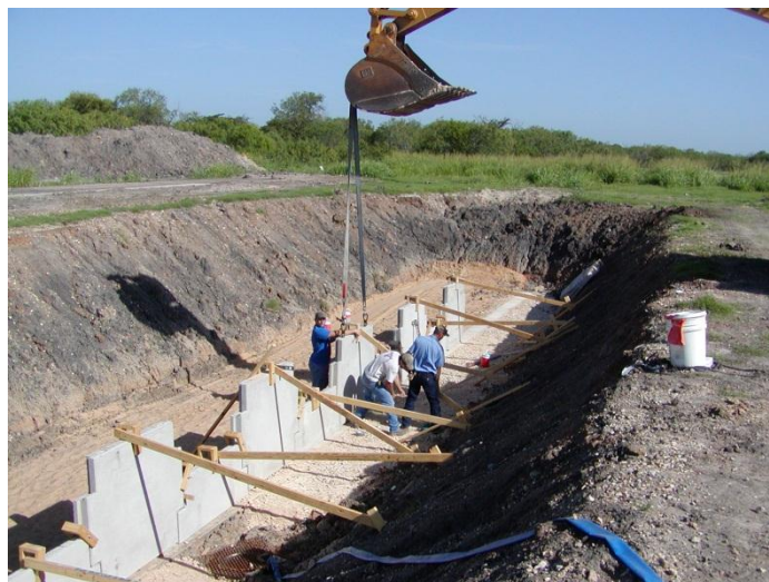
Figure D.4 Installation of the bottom layer of panels
