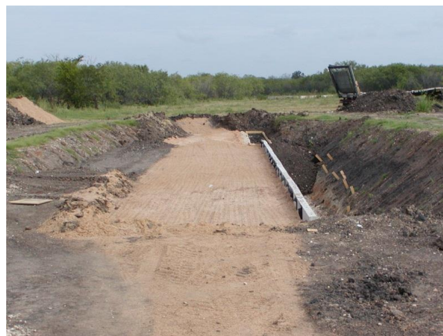
Figure D.10 Placement of the last layer of backfill material
