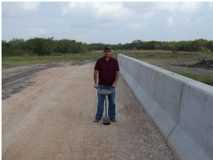
Figure D.18: BCD Modulus test in the road base material
