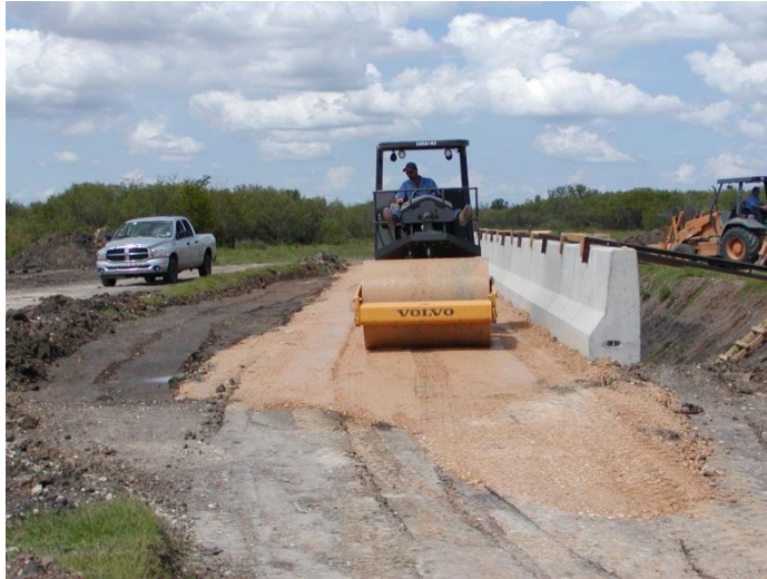
Figure D.17 Compaction process of the road base material
