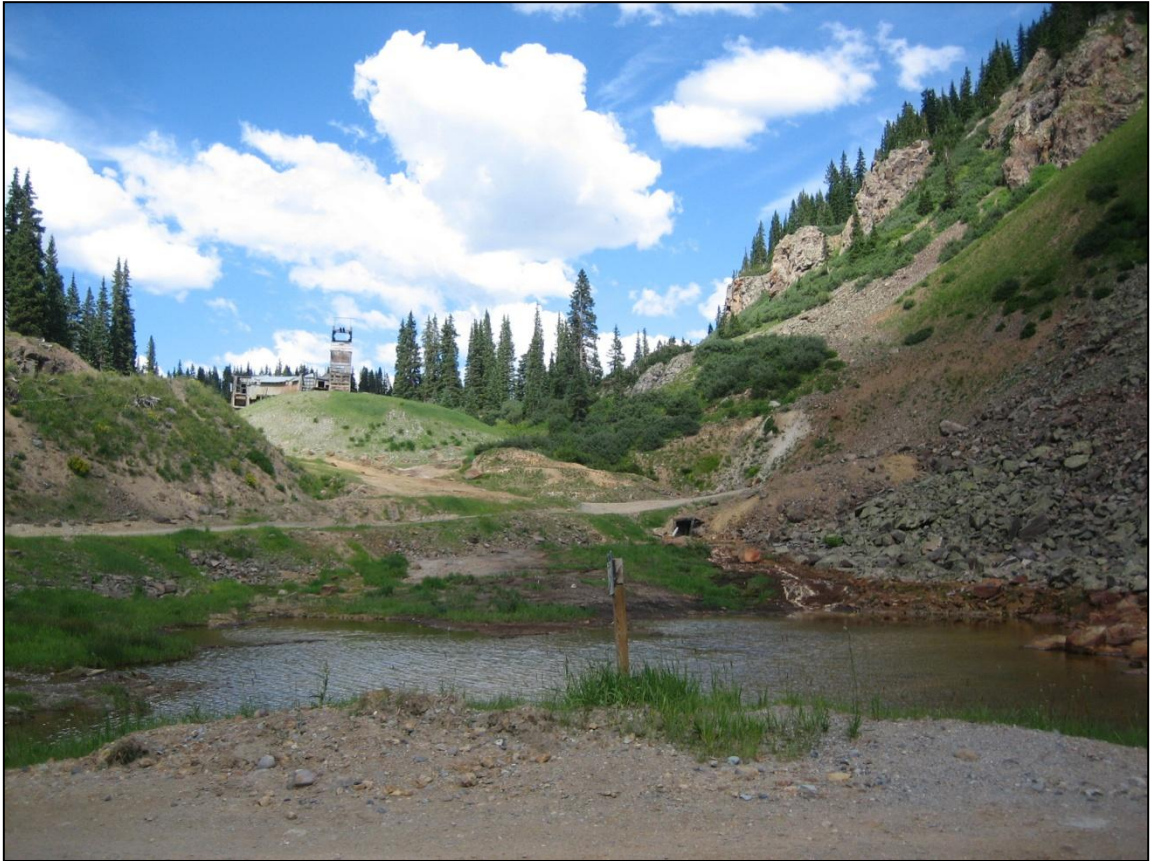
PHOTOGRAPH 6. Photograph of Longfellow Mine and a retention pond at the base of the mine and Koehler Tunnel. Photograph taken looking to the north-northeast.
