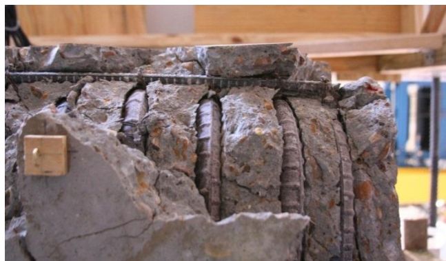
(f) Bulging of U-Shaped Steel Bars and Out-of-Plane Bending of Longitudinal Steel Bars
