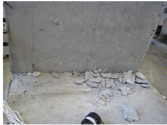
(d) Crushed Concrete at Inside Corner of Joint Region
