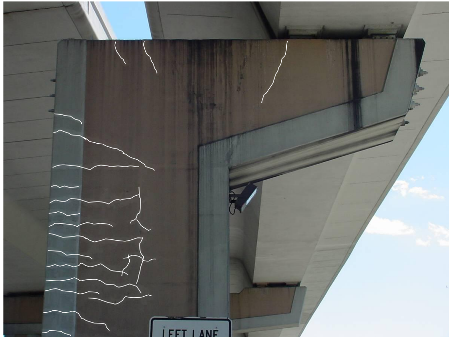
(a) Cantilever Bent (San Antonio, TX)
