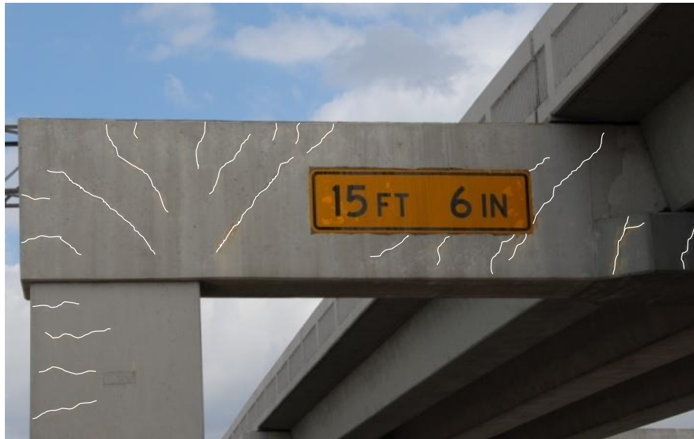
(b) Straddle Bent (Houston, TX)
