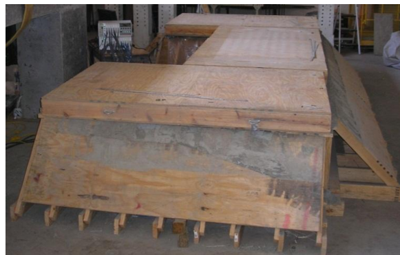
(c) ERW Panels in Position
