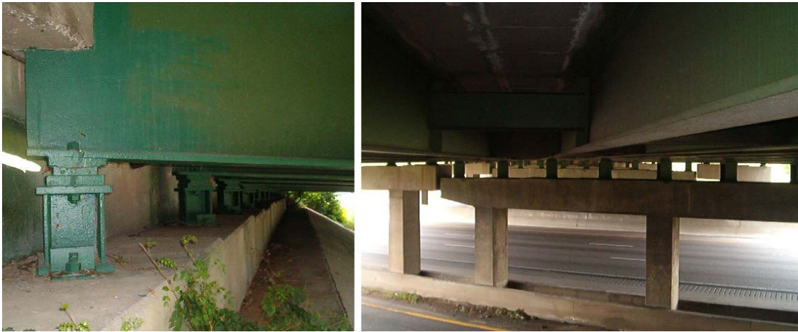
Figure 2-1. A bridge in Georgia elevated with steel pedestals
