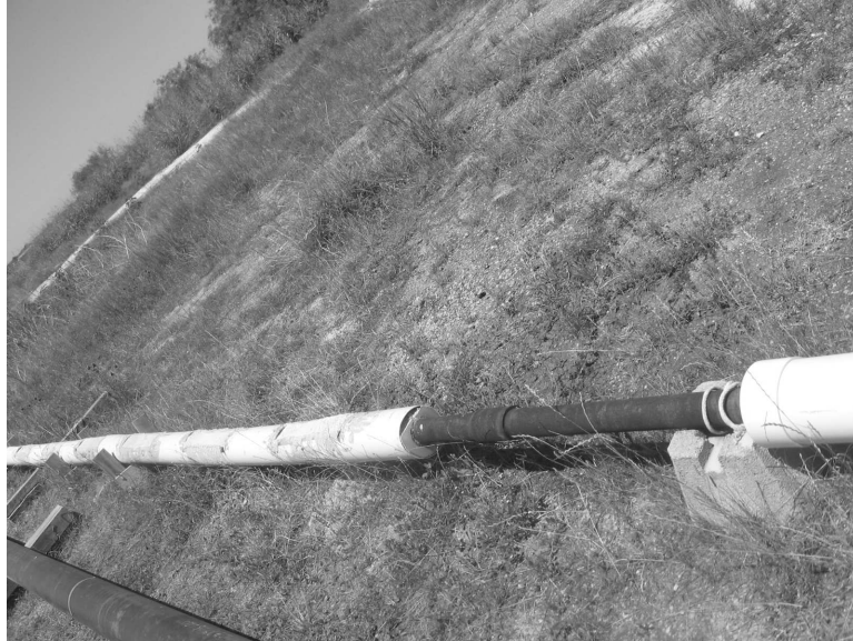
Figure 4.17: Photograph of the two concrete segments on the 2-7/8" pipe string
