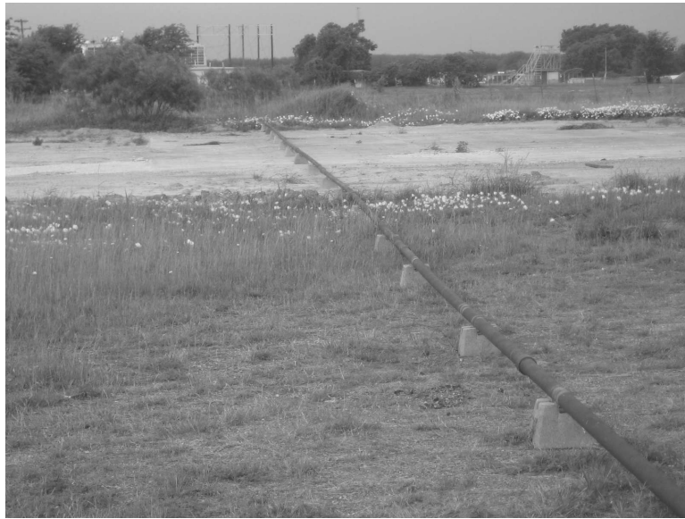
Figure 3.2: Photograph of the pipe string
