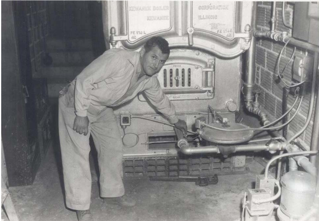
Figure 4. Mr. John and the Boiler.
