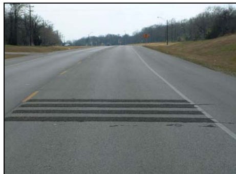
FIGURE 3 ARS Seal Coat Treatment
