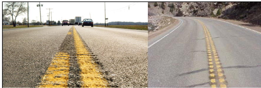
FIGURE 4 Delaware and Colorado CRS Installations
