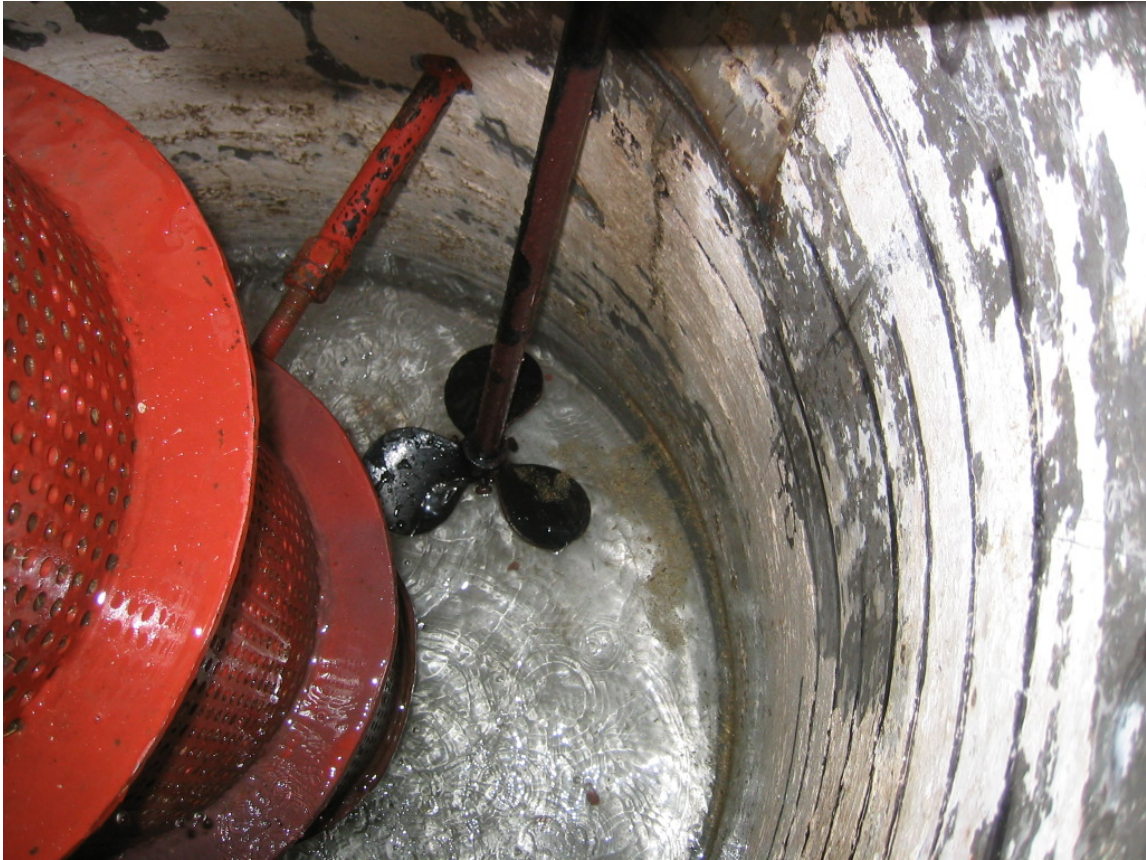
Figure 2.12 Photograph of inside the tank while being filled with water.
