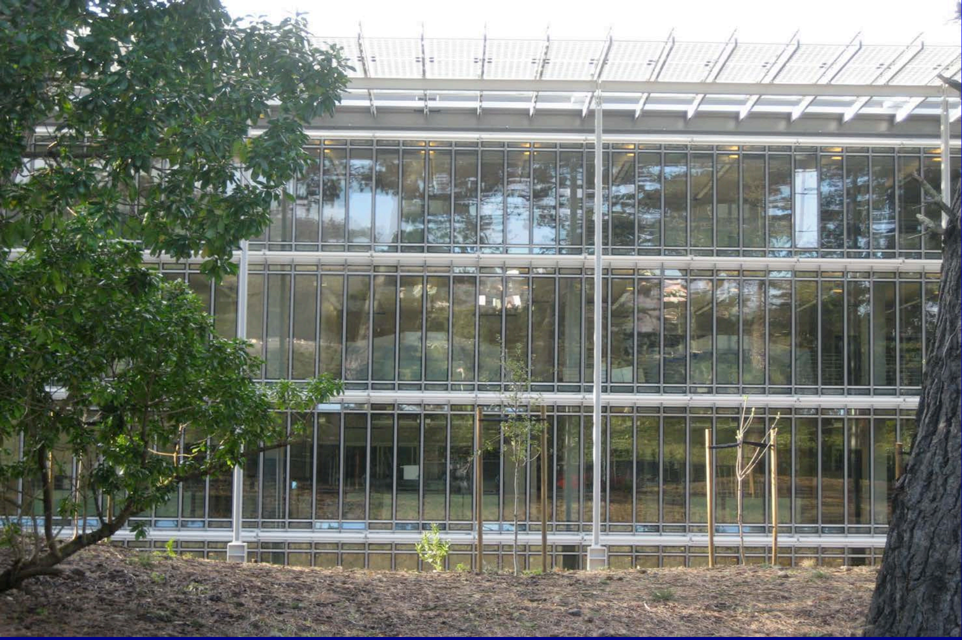
California Academy of Science Renzo Piano Architect Gartner Enclosure Center for Building Performance and Diagnostics, a NSF/IUCRC, and ABSIC at Carnegie Mellon
