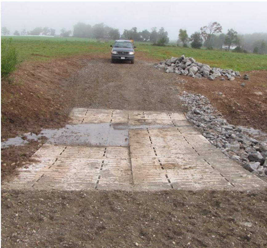
Figure 14. Hardened crossing points constructed of geotextile fabric, concrete panels, and fine gravel to facilitate cattle movement across specific points in the stream. Photo courtesy of Chenago County Soil & Water Conservation District.
