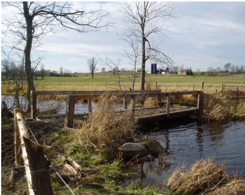
Figure 11. Above-water cattle crossing structure. Note the unaffected adjacent streambanks. Photo courtesy of Garnet Baker.
