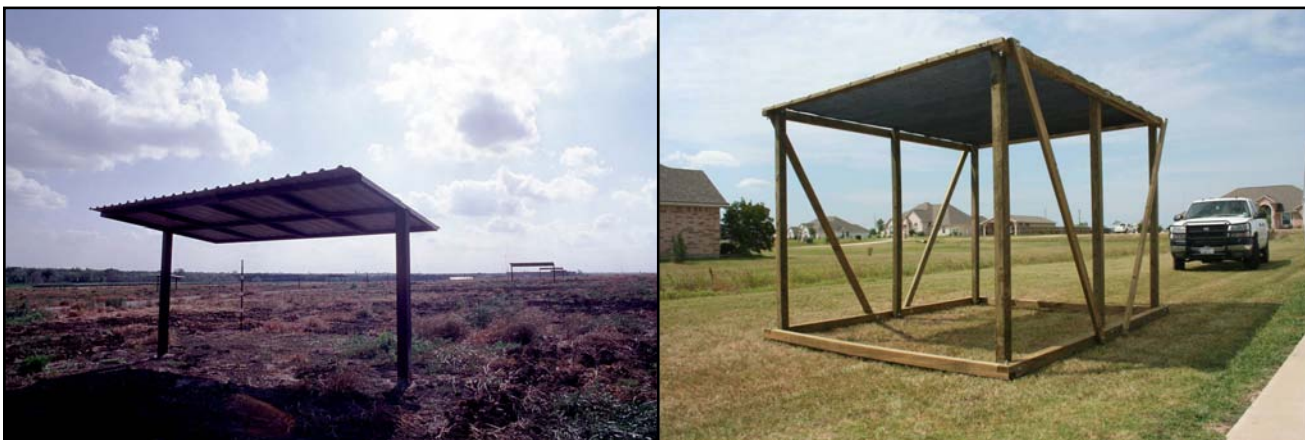
Figure 9. Shade structures constructed with a tin roof (left) and a shade cloth (right). Photos courtesy of The Samuel Roberts Nobel Foundation, Inc. (left) and Dr. Larry Redmon, Texas AgriLife Extension Service (right).
